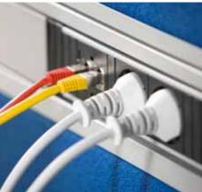
STEP is ideal for flexible power and data supply at workstations, in partition systems, false floors and other connection applications.
